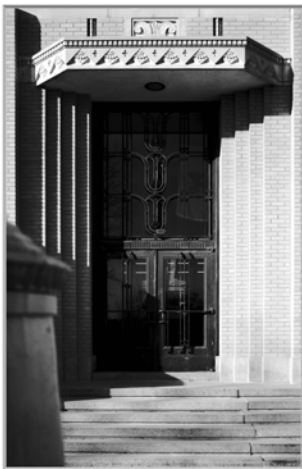
The south entrance of the Jones County Court House in Anamosa (Hughes 2009).
